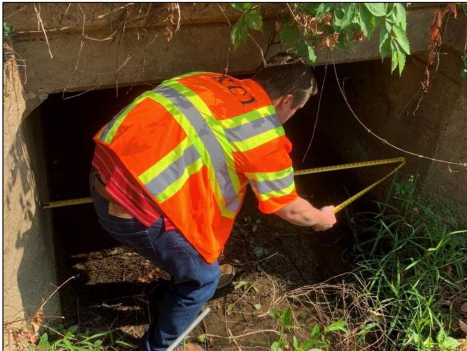
*Figure 4: Measuring width of south end of culvert @ sta. 316+23*
