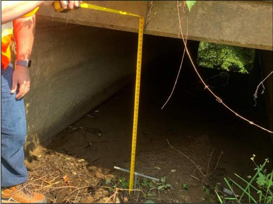
Figure 5: Measuring to top of soil at south end of culvert @ sta. 316+23
